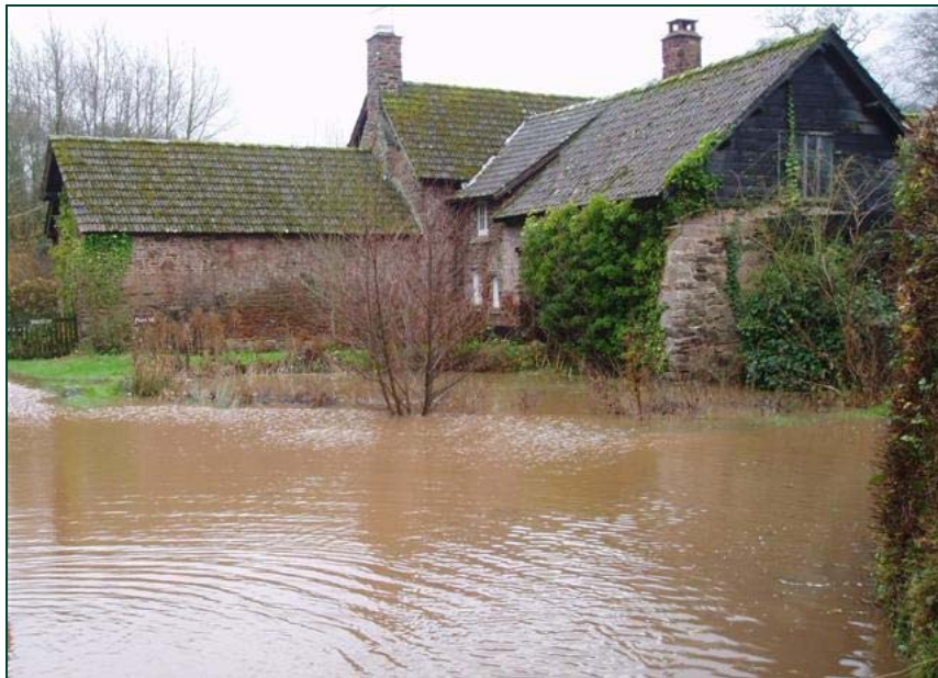
ENPA: house surrounded by flood water
