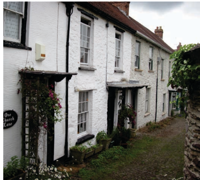
Church Terrace, small scale, rendered stone, pantile roof and pitching.
