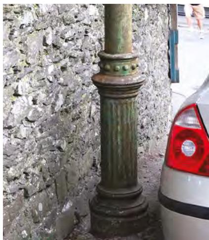
Fig 75 Sewer stench pipe.
