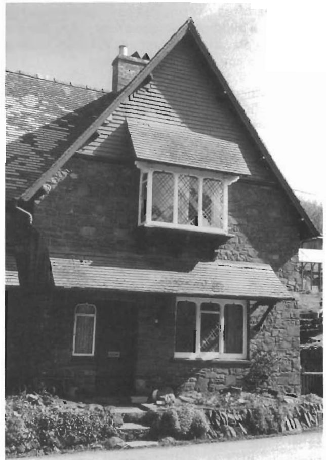
There are some buildings on Exmoor, mainly built during the Victorian period, that often display flamboyant and finely detailed features, such as these windows on a house at Luccombe.
