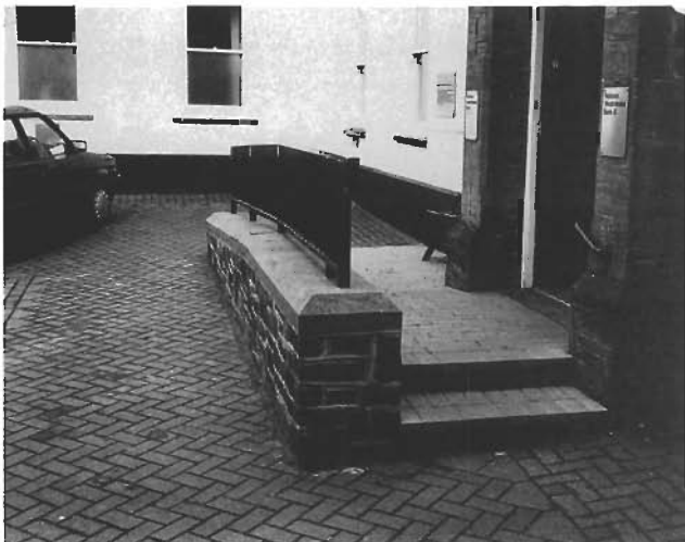
Pedestrian ramp for people with disabilities. National Westminster Bank, Dulverton.
