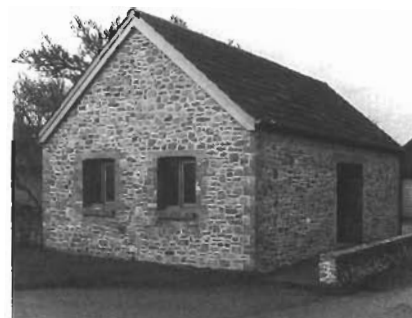
This stone built public convenience is sympathetic in both form and materials to the locality.
