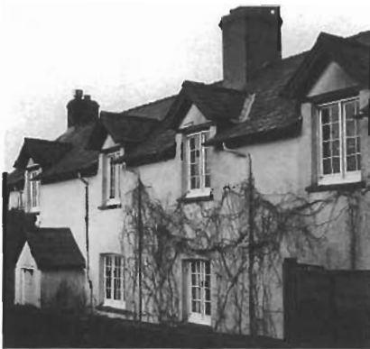
Gabled half dormers and the projecting porch provide elevational interest to this cottage in Winsford.
