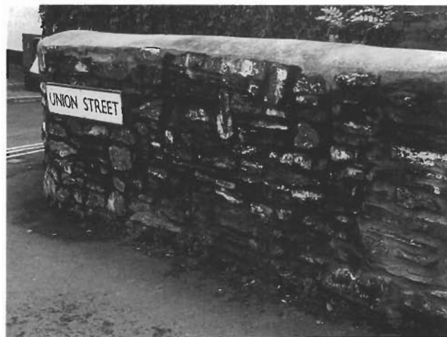
A stone wall, unsatisfactorily capped with a cement coping, readily reducing any visual qualities the wall possesses.
