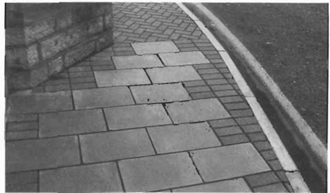
Modern concrete kerbs and small element paving. The self-conscious mixture of both materials and pattern is interesting, even if a little overdone!
