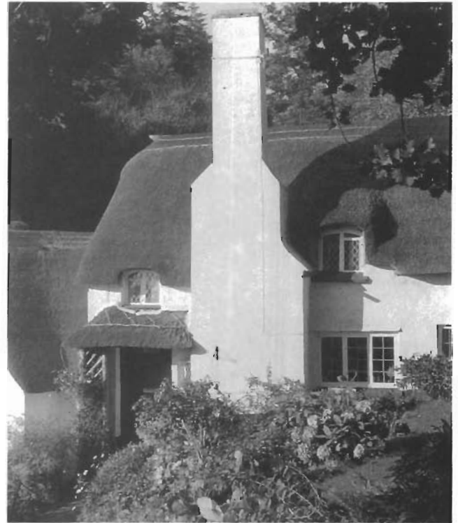
Powerful forms and soft lines typify many of the other Exmoor buildings, such as this cottage at Selworthy.
