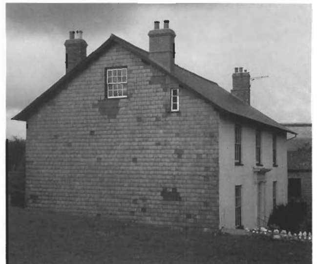
Slate hanging, is an ideal weathering face against the south westerlies, as shown on this property in Brompton Regis.
