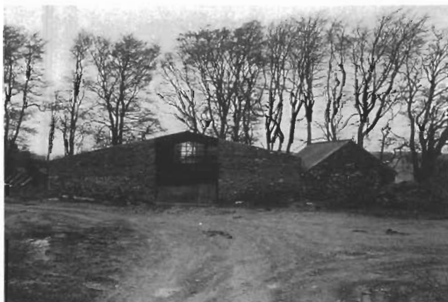
Most barns to be found on Exmoor possess strong and unpretentious shapes, well-suited to their locations.
