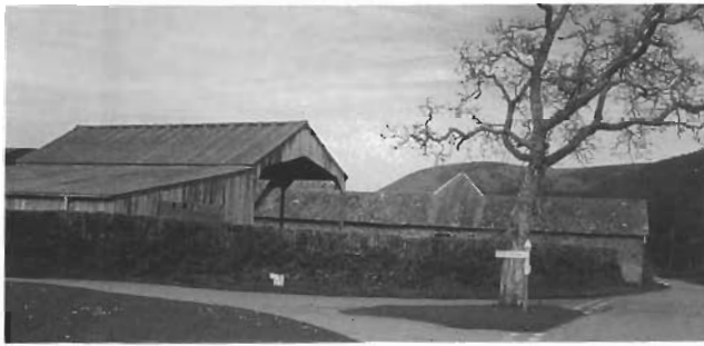
These stone barns are dwarfed by the later buildings although the lean-to in the foreground helps to reduce the effect a little.
