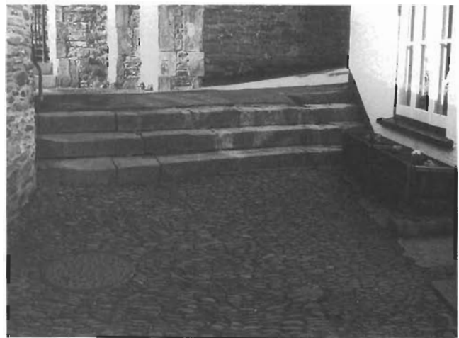
Traditional cobbled footway. Dulverton.
