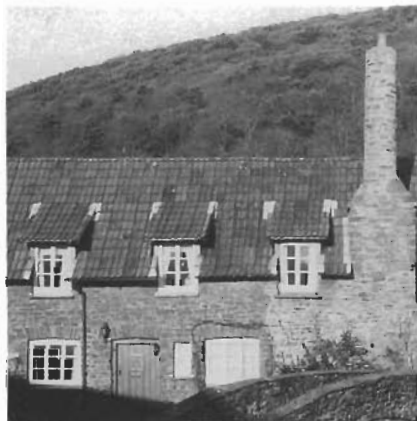
These swept dormers are a familiar sight in Allerford.
