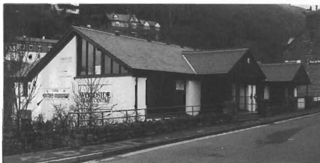
Small workshop units can often pose problems of design and scale when located within towns and villages. Here, the Woodside Craft Centre in Lymouth uses projecting gabled entrances to reduce the impact of the building in the narrow street.
