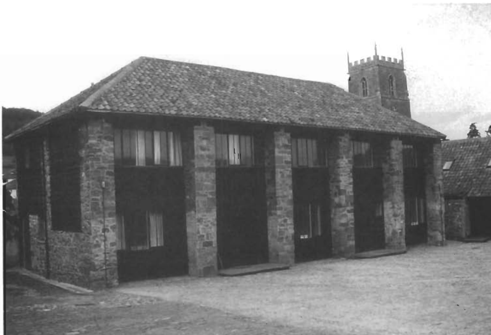
This barn at Dunster, with its columnar structure through two storeys, is perhaps not typical of barns in the region, but has been sympathetically converted into residential use while retaining the integrity of the entire building.
