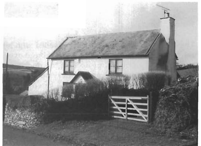
The traditional cottage design: central porch, gable-end stack and single storey outshoot can be seen in many areas of the park.
