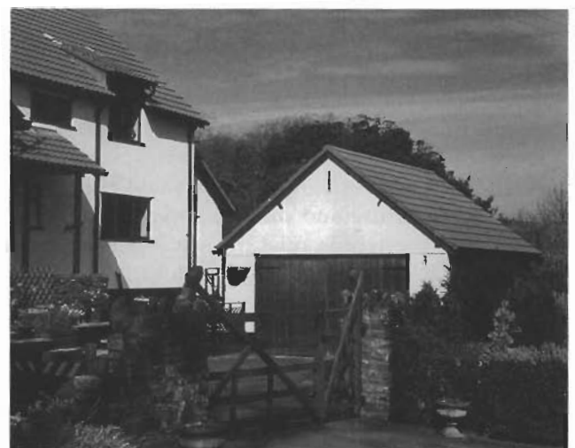
A garage placed at right angles to the main front of the house – like this example in Luccombe – may be a way, if space permits, to reduce the dominant effect such structures can have on the setting of the main house.
