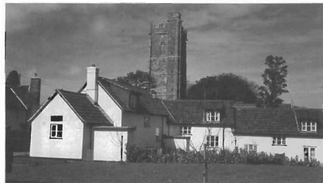
A fine grouping at Luccombe, where the West Somerset Housing Association has created, in modern terms, a successful and well-scaled terrace of houses that complements the older buildings in the village.
