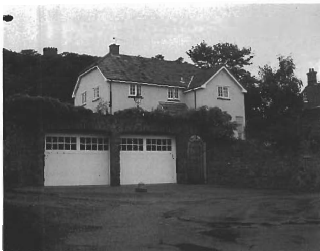
The ground levels have been used to advantage to accommodate this garage.
