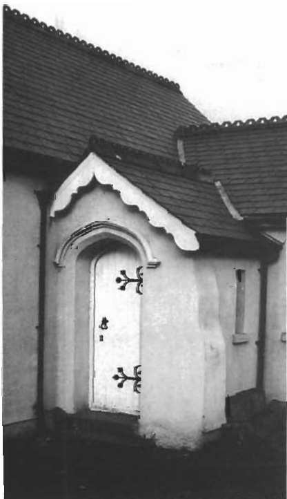
This doorway, with its pleasing stone drip moulding and ornamental fascia, has survived amidst other less sensitive restoration work.
