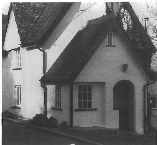
This new porch has been successfully added to an old cottage, respecting both the slope of the roof and the materials used. The use of secondhand tiles has helped considerably.
