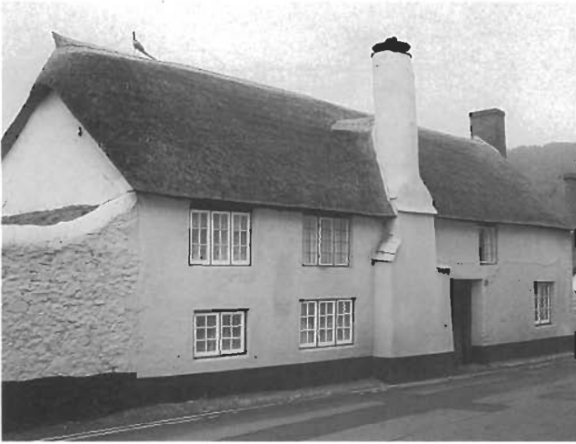
Thatch is commonly found on older buildings on Exmoor.
