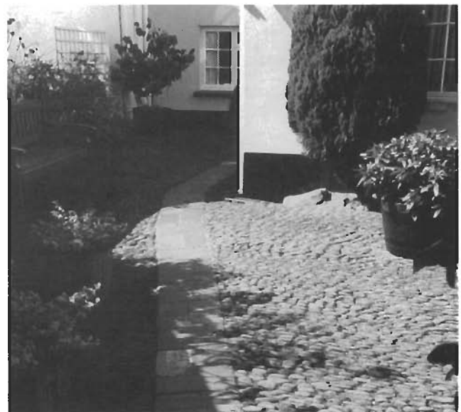
Cobbles and loose gravel are attractive but for some can be difficult to walk on. This example, within a private garden, shows what can be done to overcome this problem.
