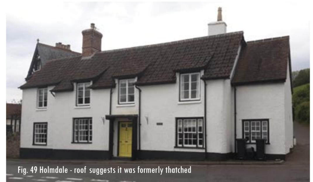
Fig. 49 Holmdale - roof suggests it was formerly thatched
