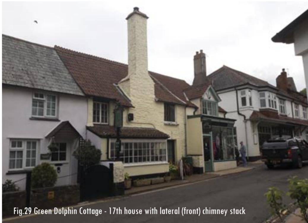
Fig.29 Green Dolphin Cottage - 17th house with lateral (front) chimney stack
