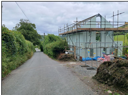
ENPA: An example of a dwelling being built in Winsford
