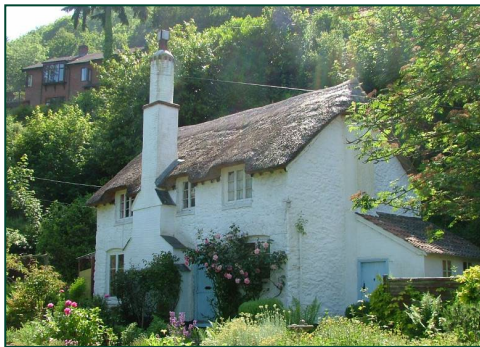
ENPA: trees surrounding cottages at Hawkcombe
