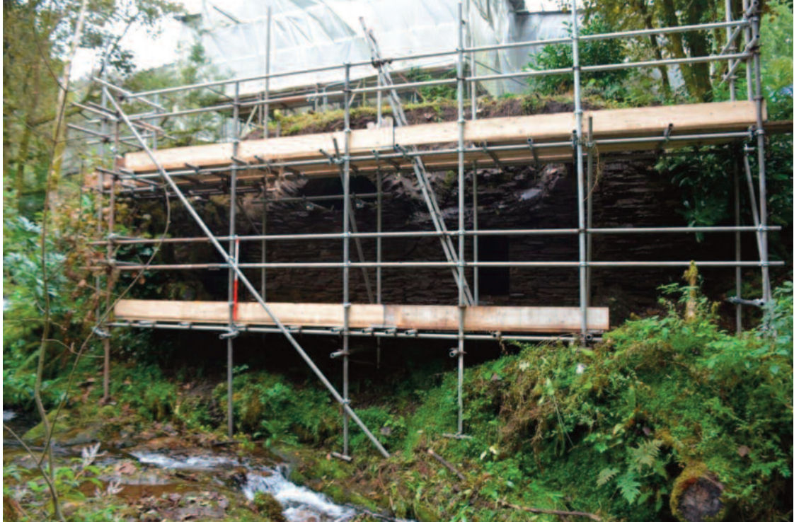
Fig. 3 The west elevation with scaffolding in place, 28.ix.16 (photo ref: SRB 9691).
