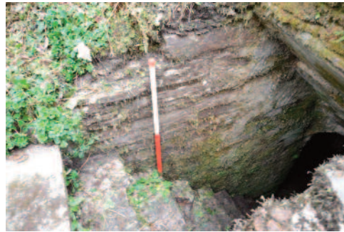
Fig. 7 East wall of stair, looking east, showing original rubble masonry throughout (photo ref: SRB 9745).
