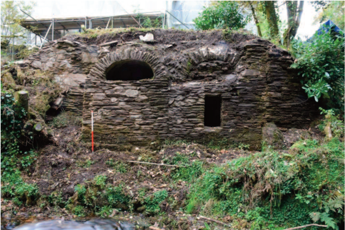
Fig. 2 The west elevation after stripping, 9.x.16 (photo ref: SRB 0037).
