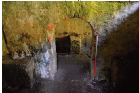
Fig. 9 Interior looking south, showing door in party wall and remains of benches in foreground and rear centre (photo ref: SRB 9563).
