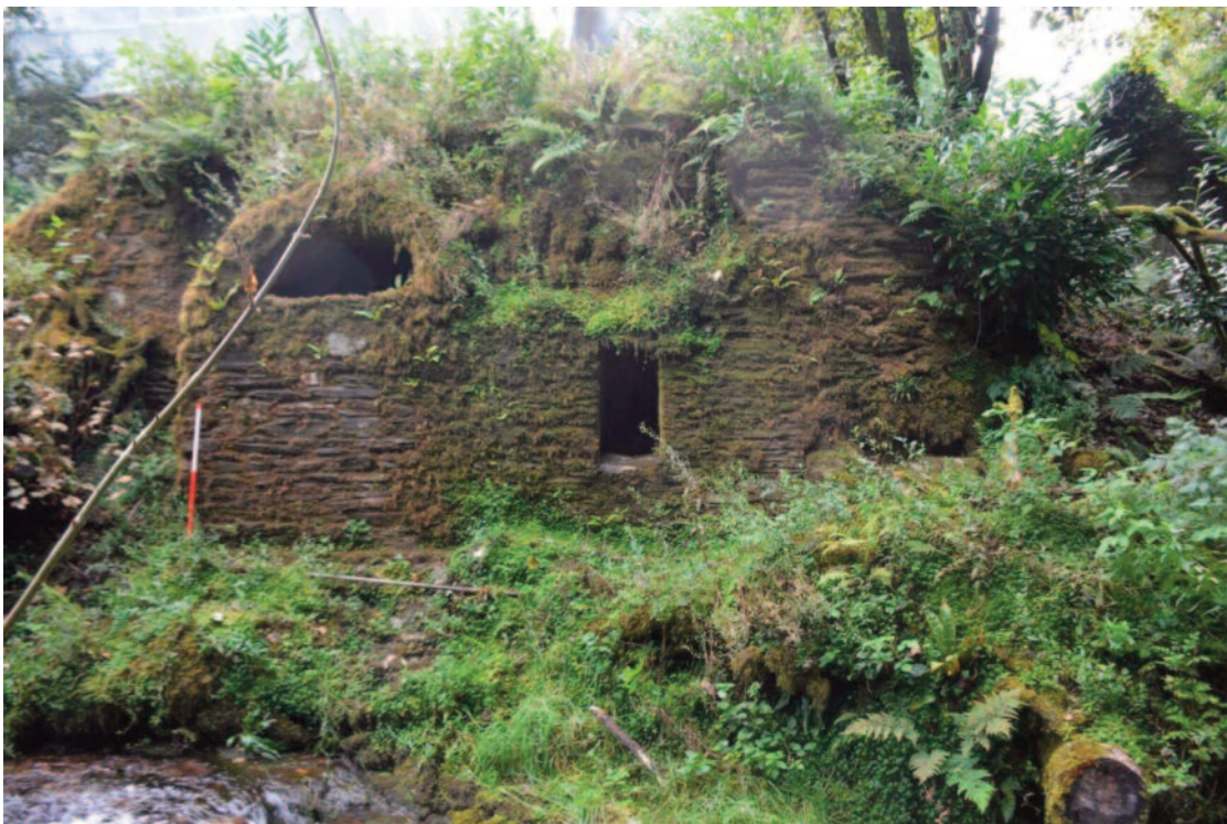
Fig. 1 The west elevation before stripping of vegetation, 7.ix.16 (photo ref: SRB 9539).
