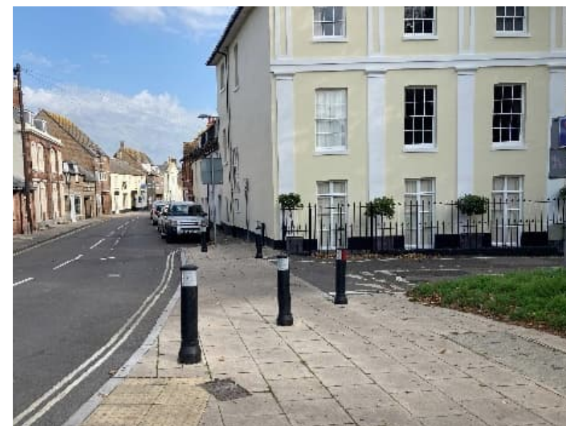
Figure 3-4 – Redesigned side road junction with greater pedestrian priority
