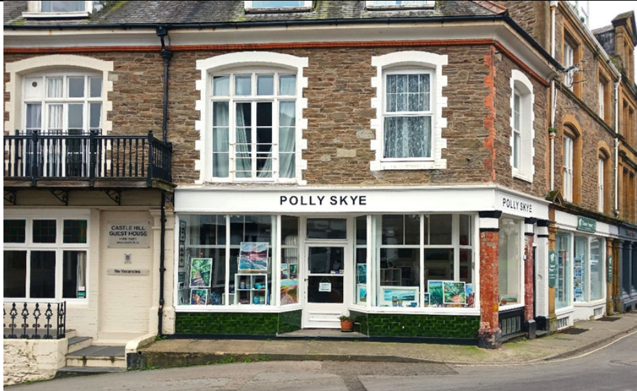
Figure 3 - Existing traditional shop frontage at Polly Skye Gallery
