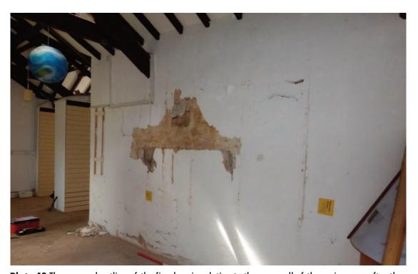
**Plate 13** The exposed outline of the fireplace in relation to the rear wall of the main range after the removal of a display panel and some paint /plaster skim.
