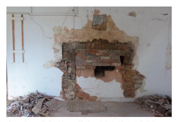
**Plate 14** The exposed outline of the original fireplace with a low brick lintel arch after further opening up. Note the strip of brick infill on the left jamb showing narrowing, the partially exposed stone floor or hearth and the slate panel 0.30m x 0.30m centrally placed above the fireplace.
