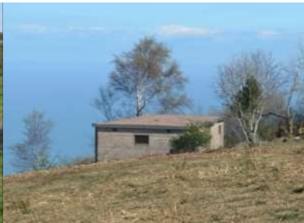
Figure 10: North Hill radar station after conservation works
