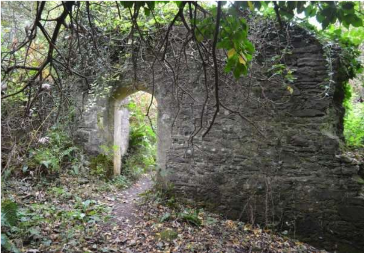
Figure 115: Burgundy Chapel, showing vegetation coverage of the monument
