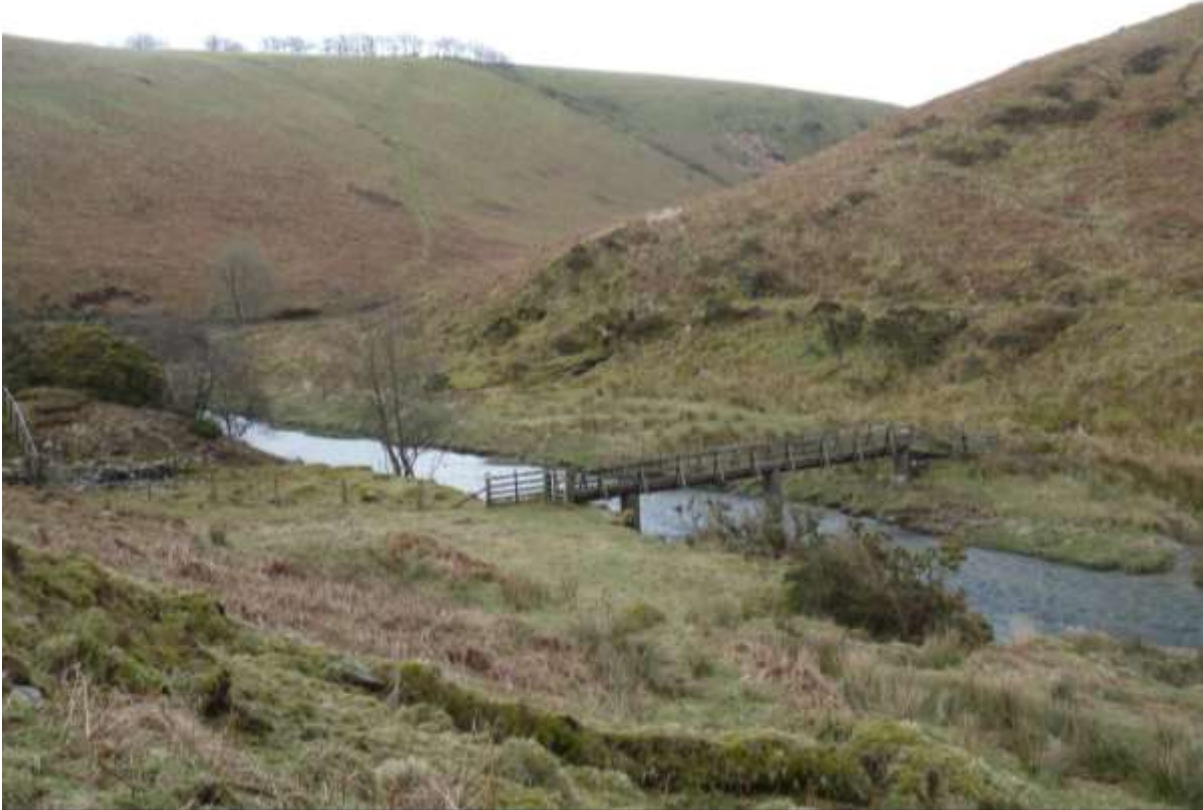
Figure 113: Looking back into the PAL from the east, mine shafts and workings are visible at the far left of the image (Photo: ENPA)
