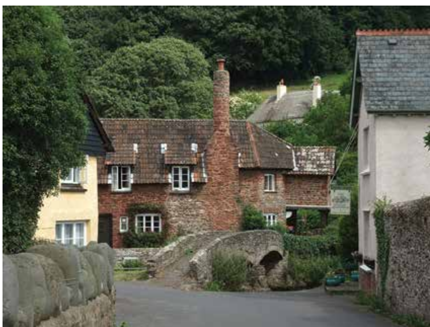
Fig. 11 View to the packhorse bridge from south.
