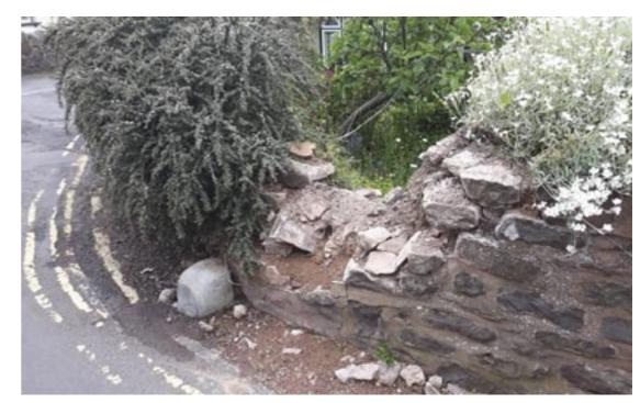
Fig. 78 Damage to wall presumably cause by vehicles
