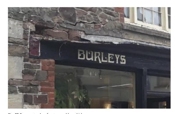
Fig. 79 Damage to shop front caused by vehicle
