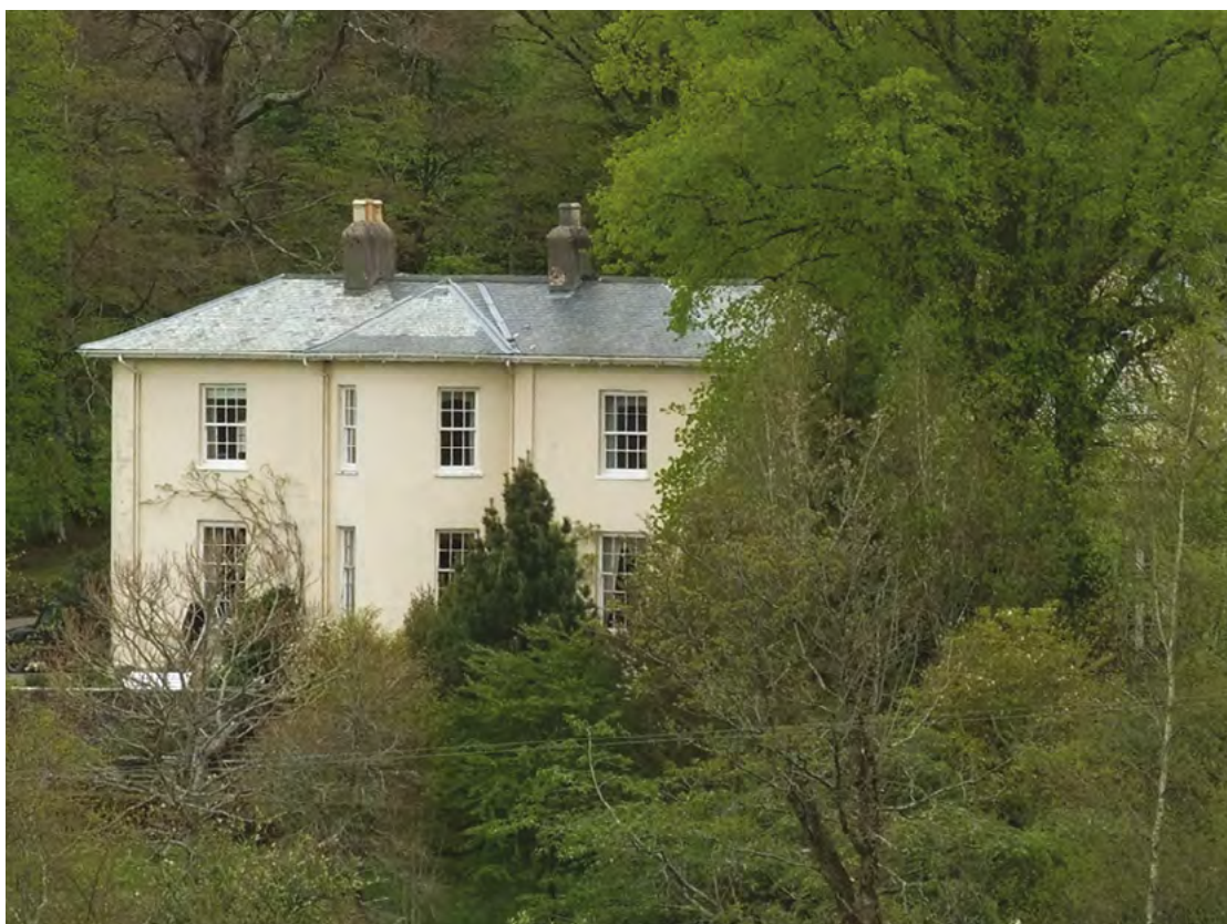
Fig. 31 South front of Heddon Hall.
