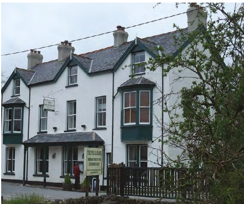
Fig.12 Fox and Goose public house – late nineteenth century façade.
