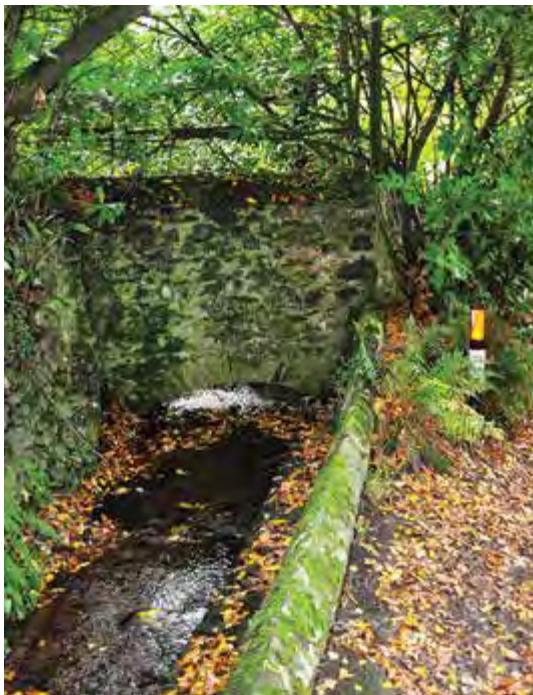
Fig.40 Access bridge off main road
