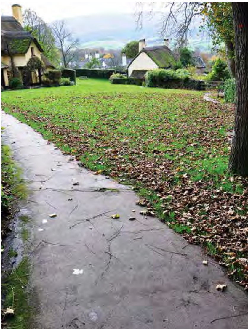
Fig.44 Tree root damage to path on the Green
