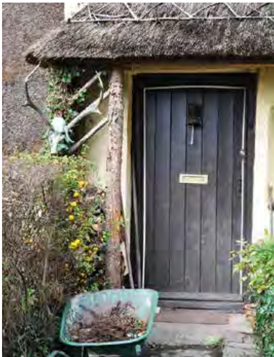
Fig.13 Rustic porch detailing, Postman's Cottage
