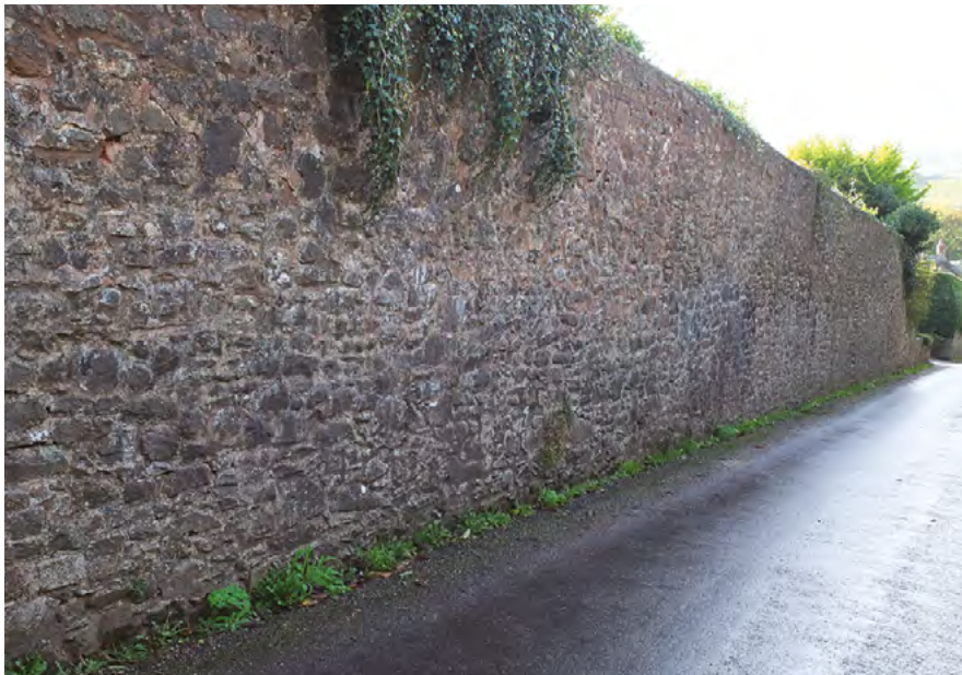
Fig 35 Boundary wall to Old Rectory
