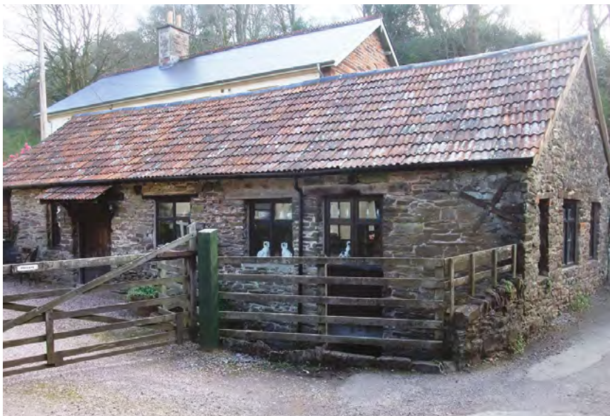
Fig. 58 Former Smithy, wheel pit with remains of wheel to the left.
