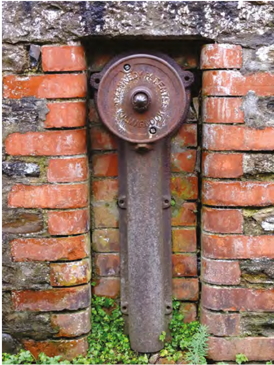
Fig. 82 Water hydrant, Church Lane
