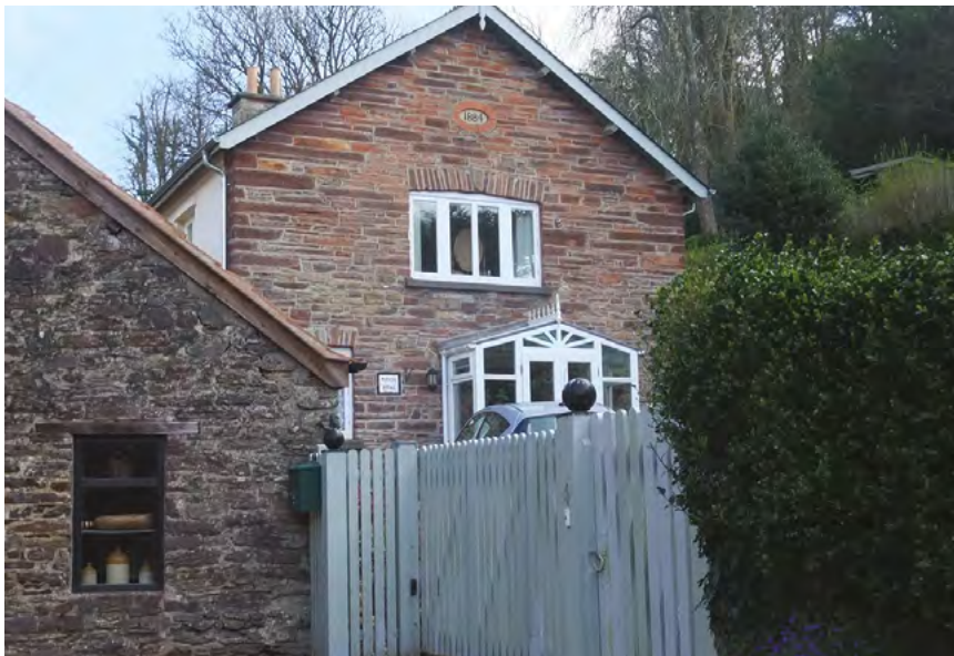
Fig. 57 Former Plymouth Brethren Chapel, now dwelling.
