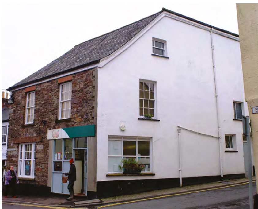
Fig. 25 Dulverton Post Office, corner of High Steet and Lady Street
