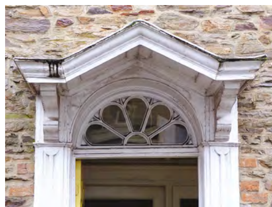
Fig. 77 Fanlight at Billbower House
