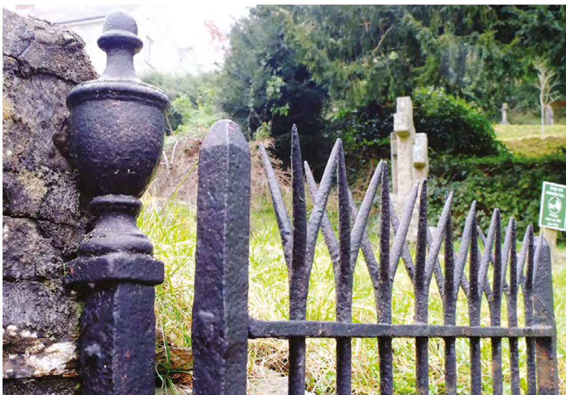
Fig. 79 Part of the ironwork surrounding the church.
