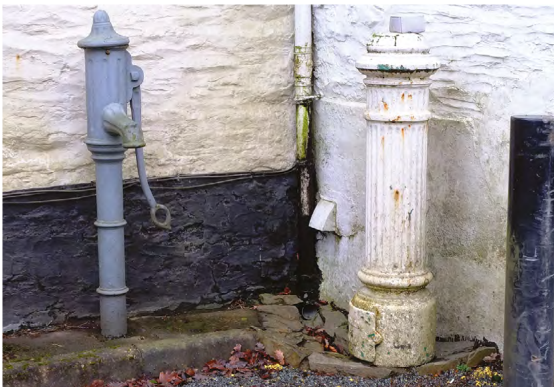
Fig. 81 Bollard and hand pump at Northmoor Road
