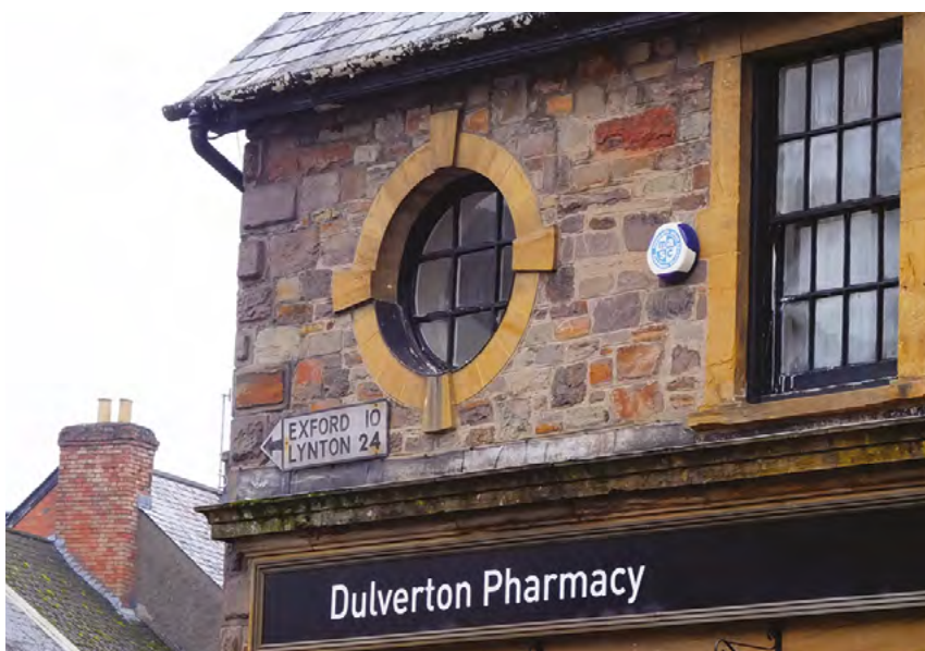
Fig. 33 First floor roundel window to Dulverton Pharmacy.
